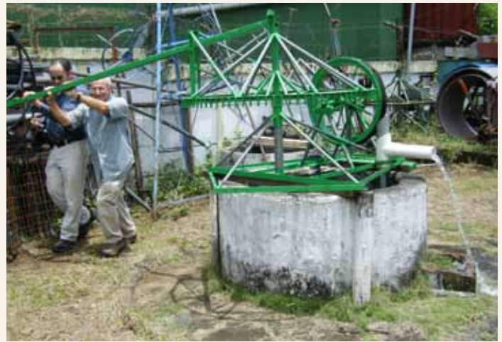
Ahmed Amer and Jim Reites, S.J., operate a rope pump system in Nicaragua.
