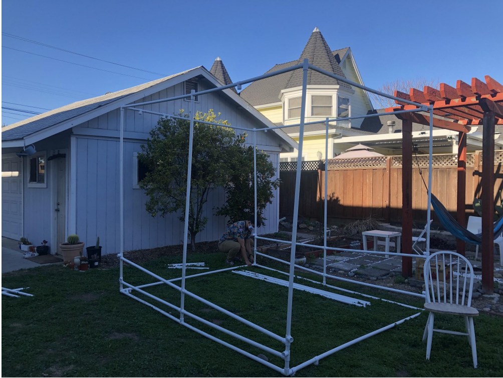
Figure Q-3: Vent Walls Connected and Upright
