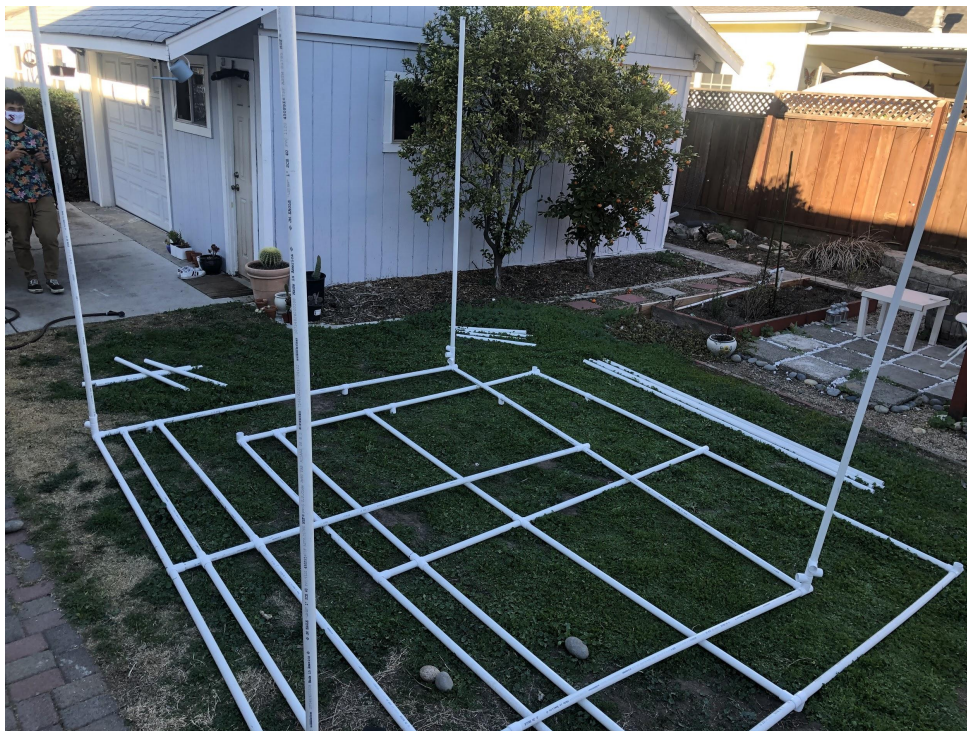
Figure Q-2: Two Vent Walls, Support Posts and Fittings Attached
