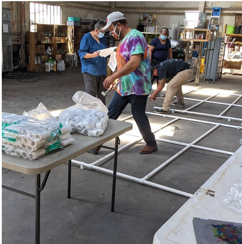
Figure 5.8: Super Jardineros collaborating to construct the first two walls of the greenhouse
