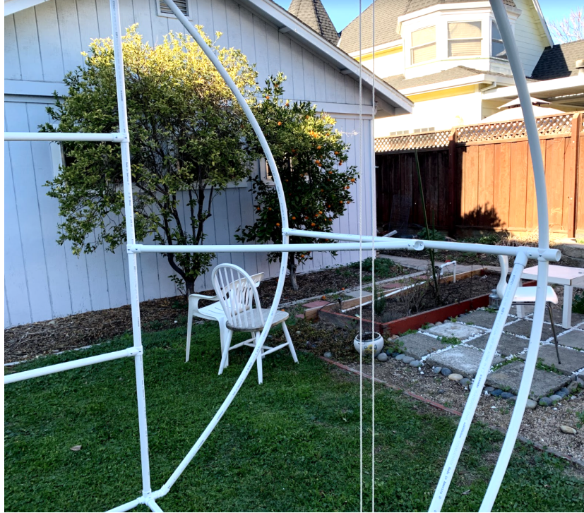
Figure 5.2: Close up of diagonal roof supports
