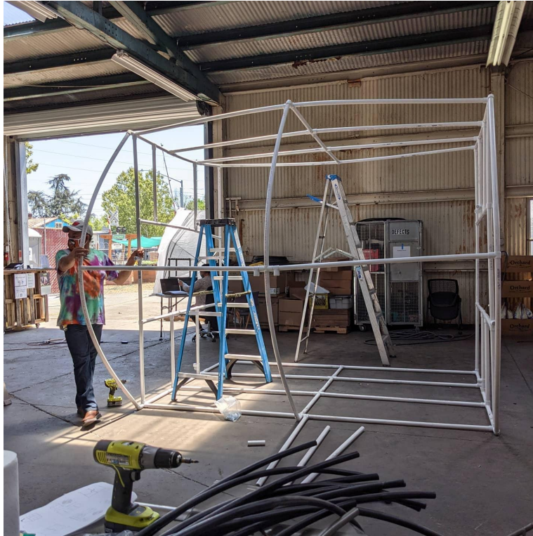
Figure 5.9: A Super Jardinero standing next to the partially completed greenhouse
