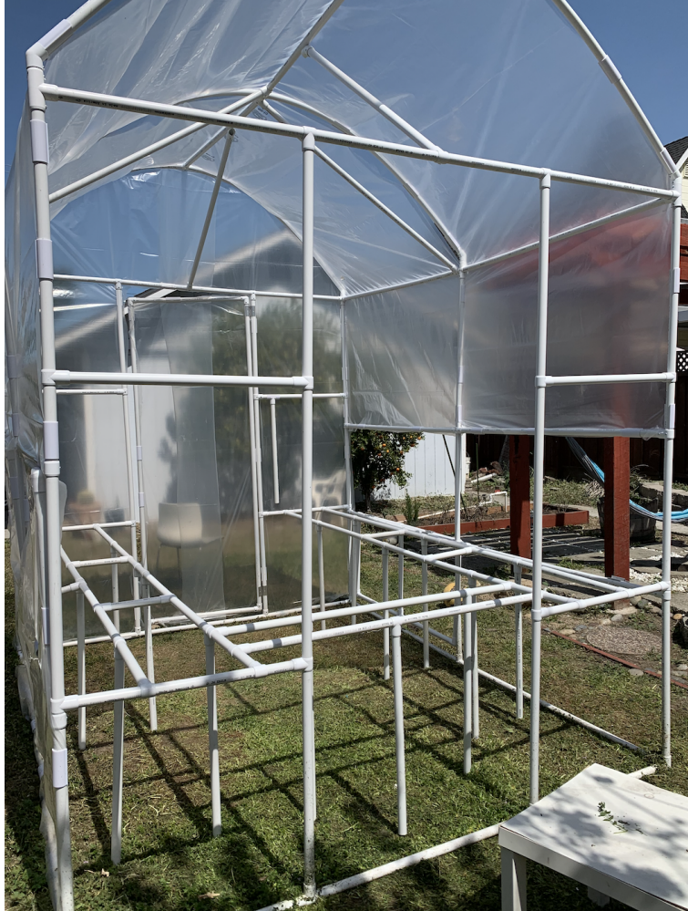
Figure 5.3: Greenhouse with Five Foot Wide Plastic
