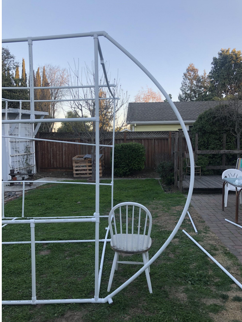
Figure Q-5: Greenhouse Turned Sideways, Domed Roof Beam Added (10' length shown here)
