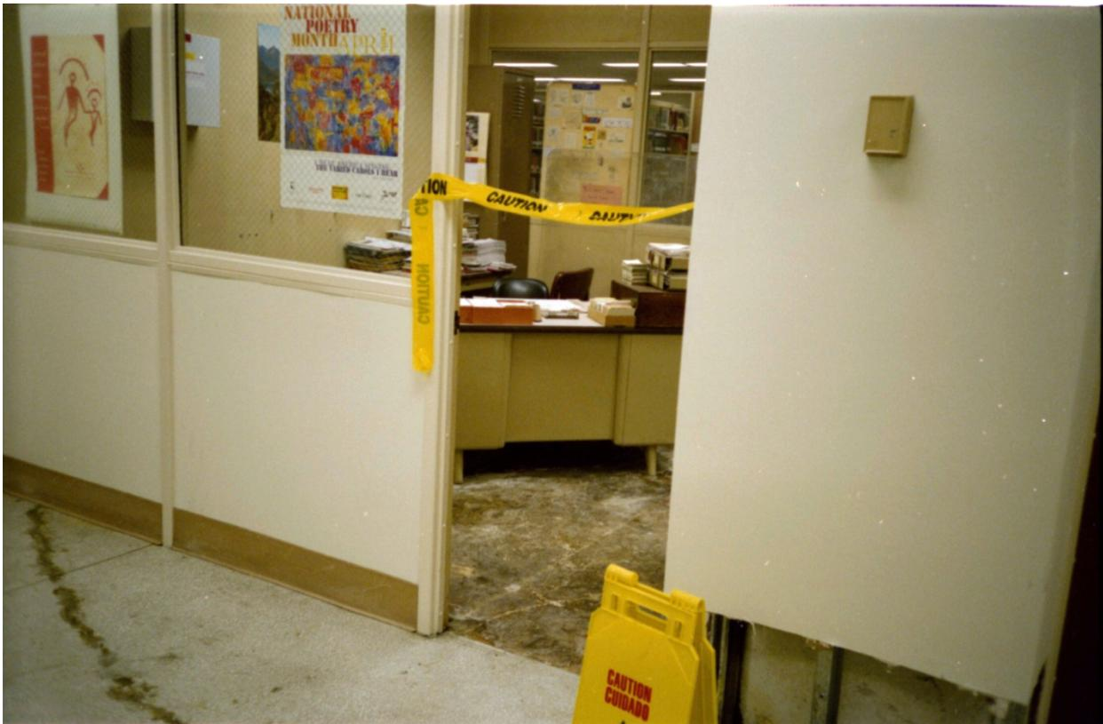
Photo #2. The exposed concrete slab shows widespread fungal growth and water damage in this view looking into the same office. Across the lower left corner of the photo, groundwater can be seen seeping up through a crack in the terrazzo floor outside the office.
