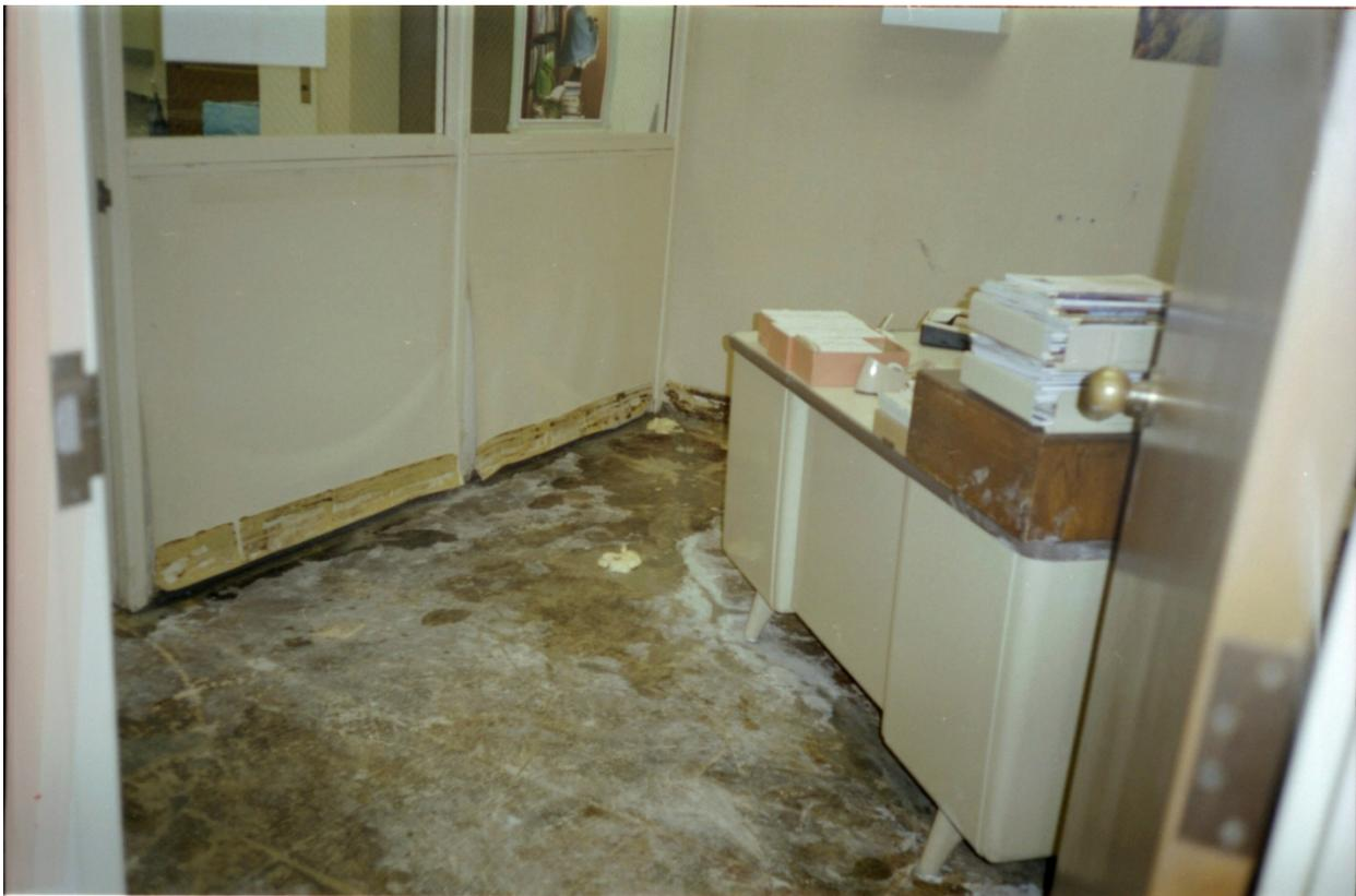
Photo #1. This office, which was identified as an "amplification site" for *Penicillium* and *Aspergillus* molds, shows how extensive the damage was. Dirty brown standing groundwater and white mold discoloration can be seen all over the floor. The bright cream-colored globs are the silicone substance that was originally injected into leaks to stanch the flow of water. Damp wallpaper is curling up away from where damaged baseboards have been removed.
