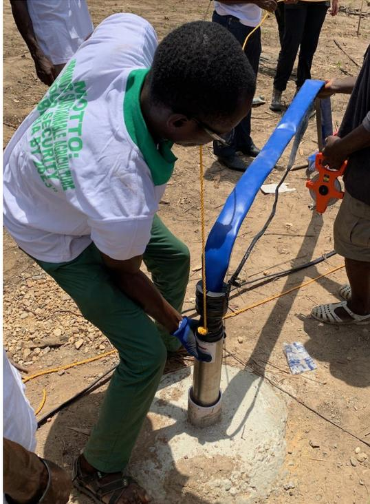
*Figure 7: The pump connected to the blue discharge pipe, the yellow safety cord, and the black power cord.*
