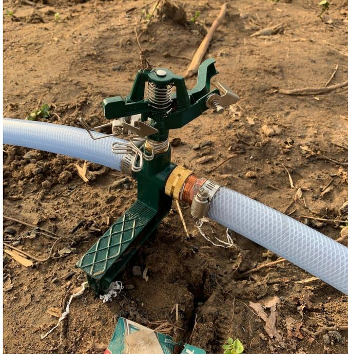
*Figure 11: The connection of the sprinklers to the mainline using male and female adapters.*
