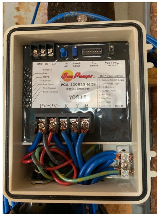
**Figure 10:** The wiring that connected the solar panels and pump, and the controls of the pump's flow rate.
