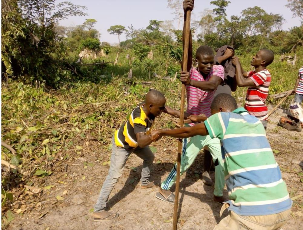
*Figure 8: Well contractors hand drilling the constructed well near Janzon Town.*
