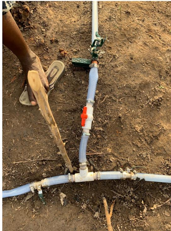
*Figure 12: The connection of valves to the hose at a T-joint using male adapters. Valves can be seen on all three sides of the T-joint.*
