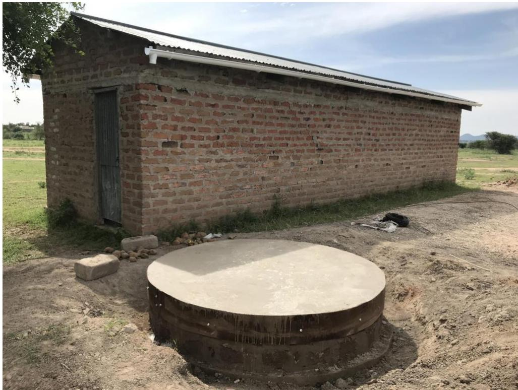
Figure 13: Finished non-potable tank foundation in the process of curing.
