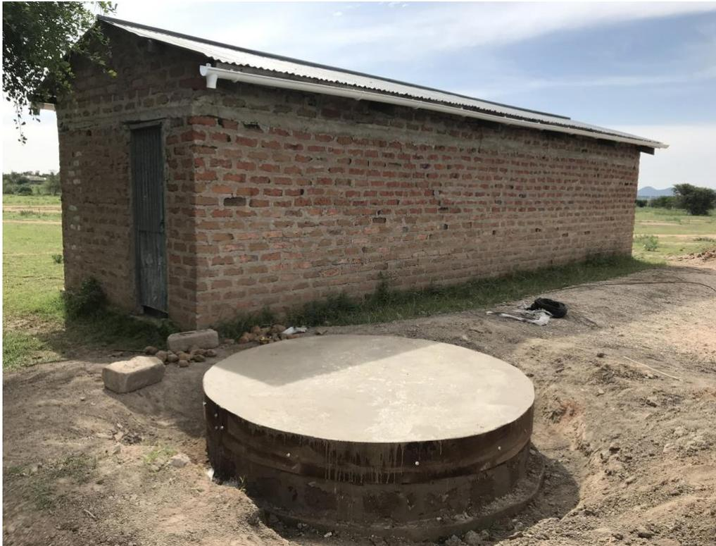
Figure 13: Finished non-potable tank foundation in the process of curing.
