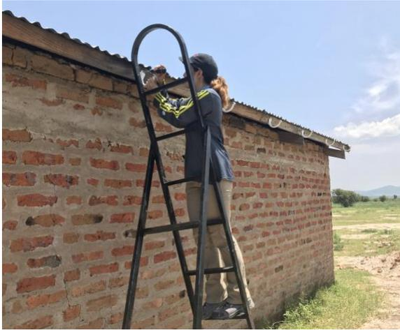
Figure 11: Plastic gutters snapped into place.
