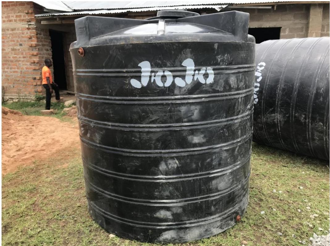
Figure 14: 10,000 L tank with brown ¾" gaskets installed at the top and bottom of the tank.
