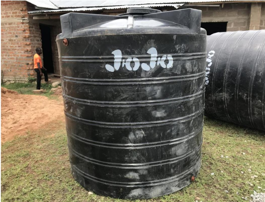
Figure 14: 10,000 L tank with brown  $\frac{3}{4}$ " gaskets installed at the top and bottom of the tank.
