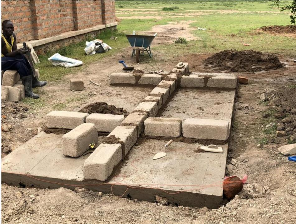
Figure 12: First layer of brick for the cross foundation.
