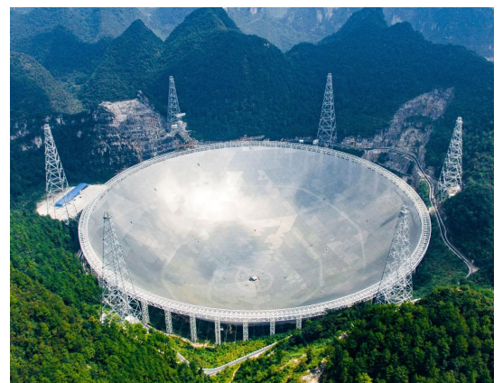
FAST radio telescope located in southwest China. Is the one of largest single aperture telescopes in the world. The dish itself has a diameter of 500 meters.
