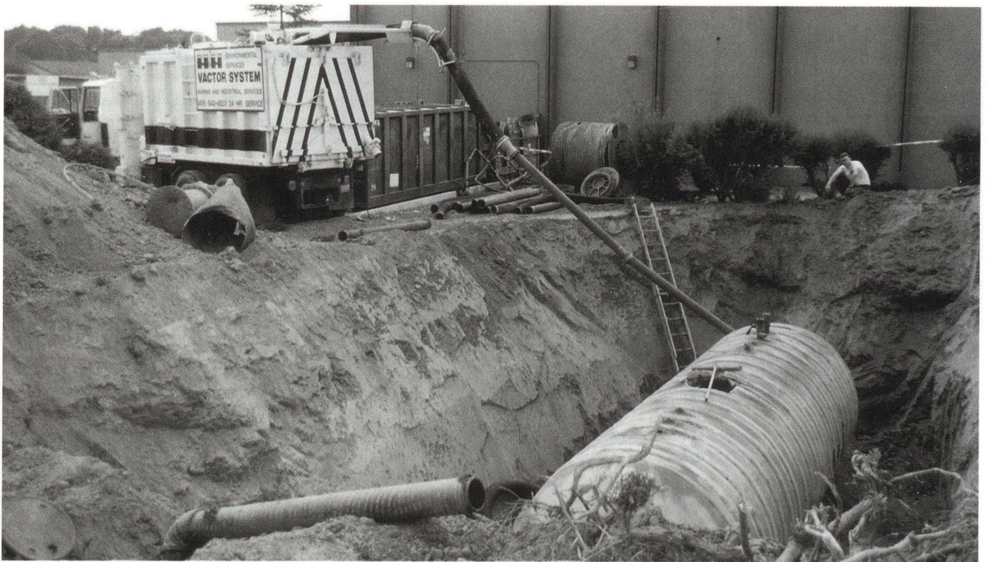
HSR removes an underground oil tank from a local high school
