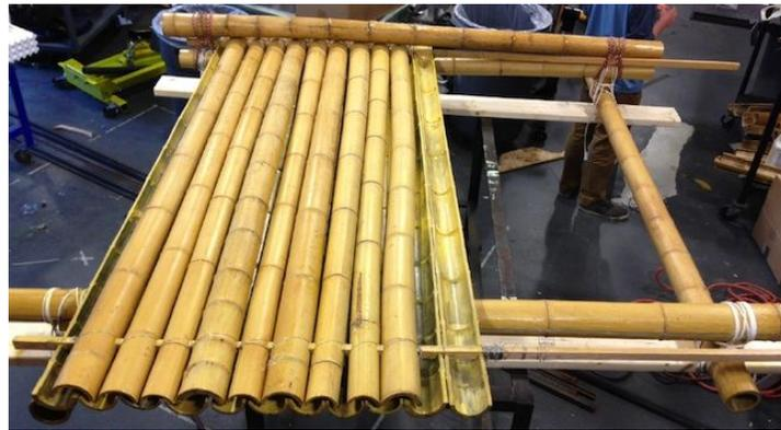
**Figure 2: Initial roofing design possibility using bamboo.**
