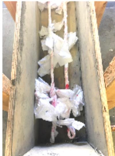
**Figure 8: The plastic grocery bag rods set into the formwork.**
