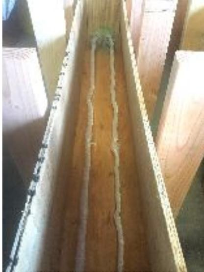
**Figure 9: Fish netting rod set into the formwork.**
