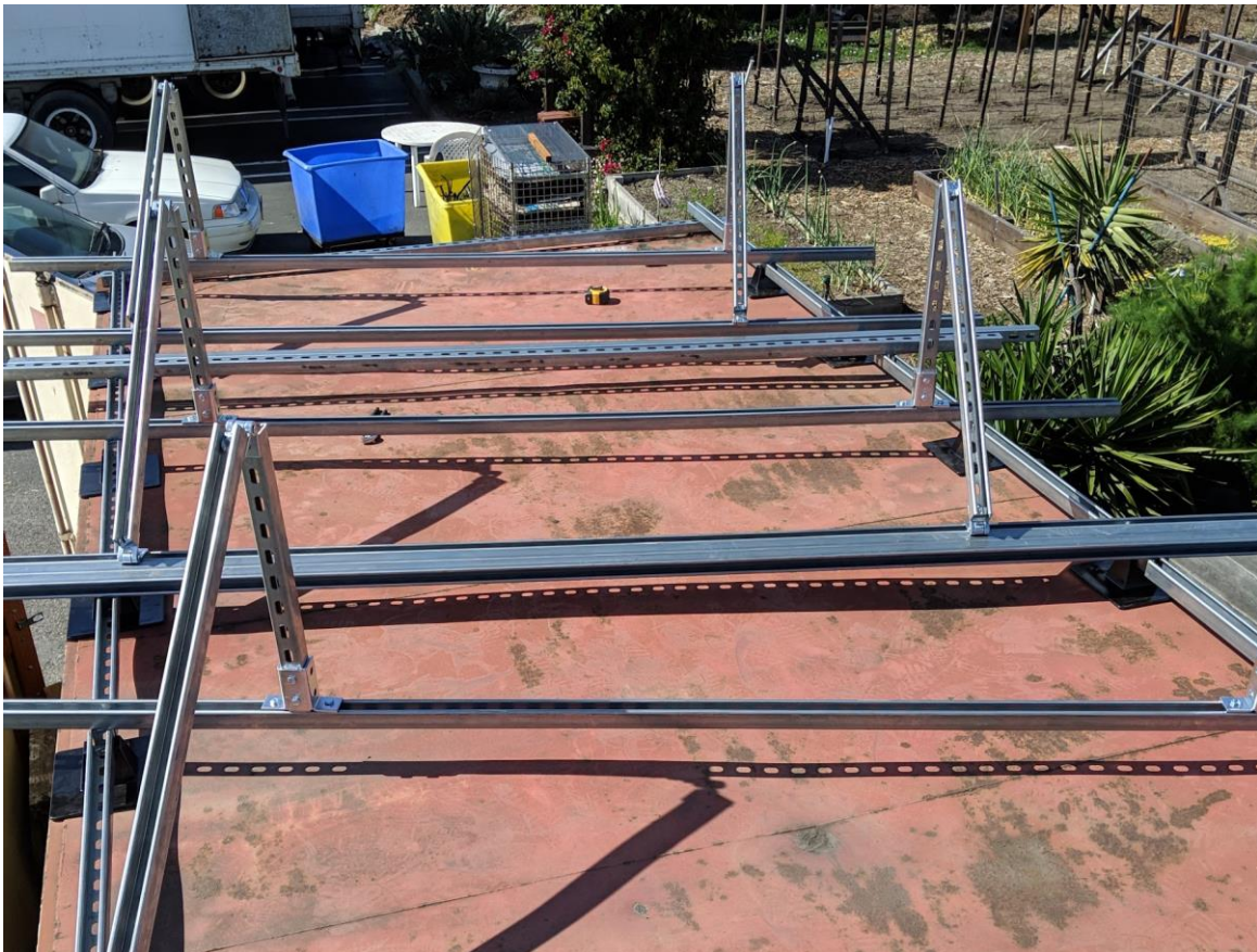
Figure 40. Completion of step 3, attaching the triangular frames
