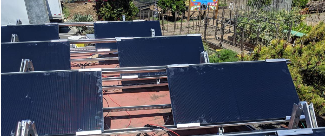
Figure 43. Mounted solar panels with the end clamps
