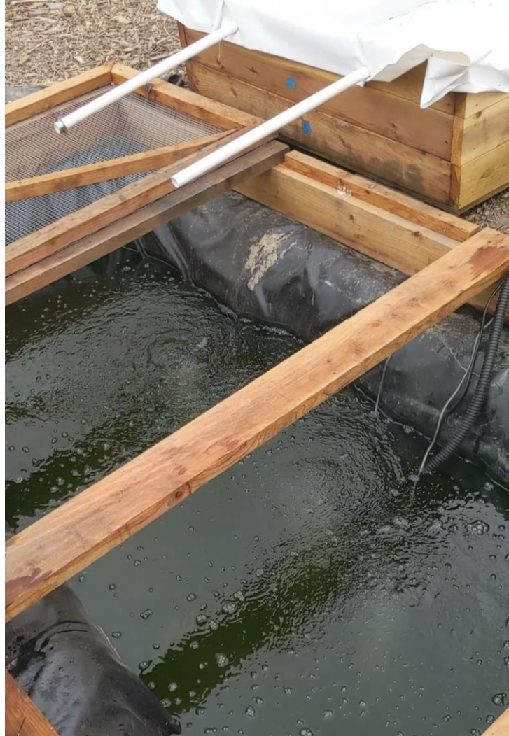
Figure 19. Completed pond with cover, aeration, and fish
