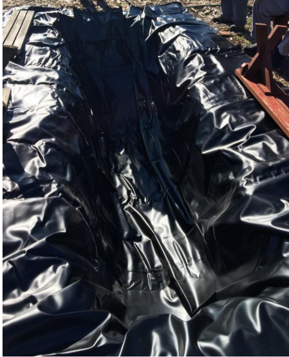
Figure 15. Empty fishpond with underlayment
