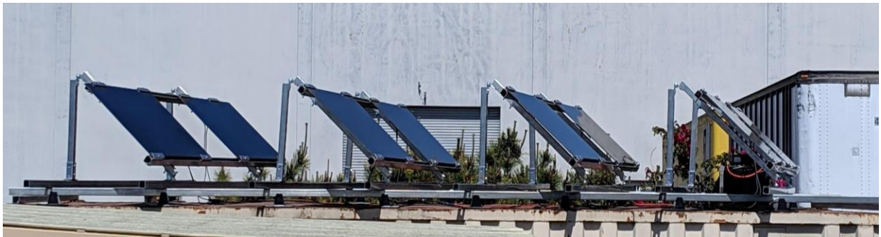
Figure 44. Side view of completed solar panel system
