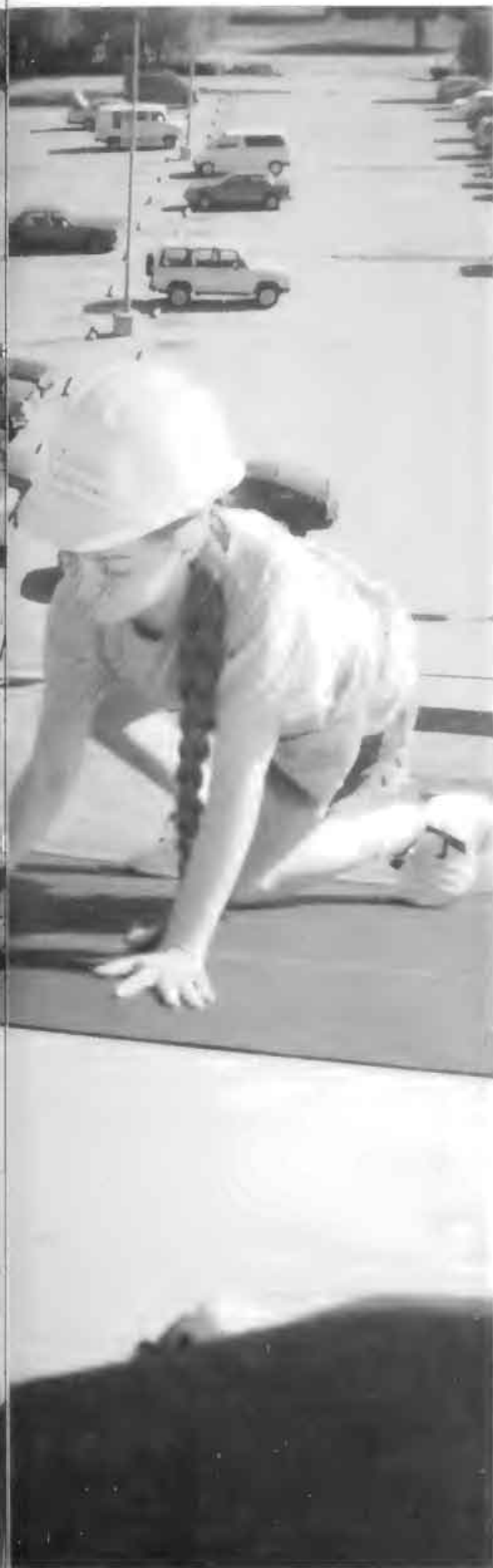
S enior Amy Koenig tacks tar paper to a roof for Habitat for Humanity. Habitat is sponsored by Campus Ministry throughout the year as an alternative spring break trip. (Left)
