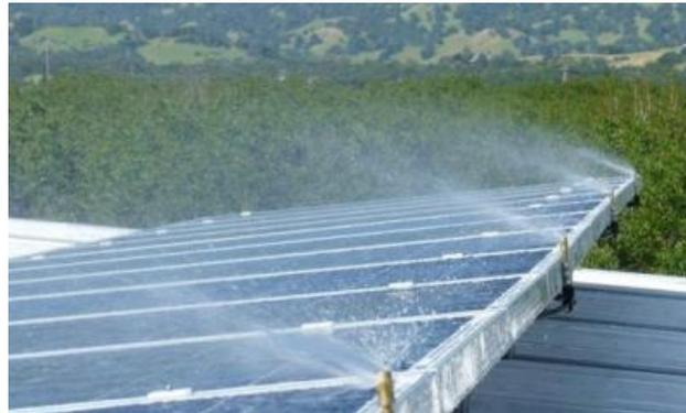
Figure 6: Heliotex sprinkler system<sup>8</sup> (Reproduced without permission)
