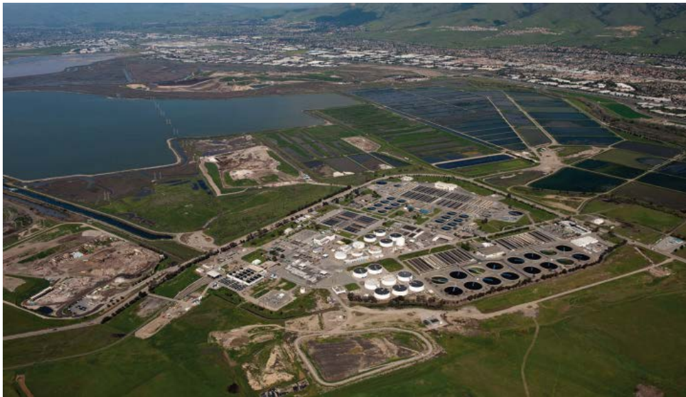
Figure 1: Aerial photograph of the Regional Wastewater Facility
