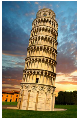
Figure 1: The Leaning Tower of Pisa, a popular case study in foundation settlement
