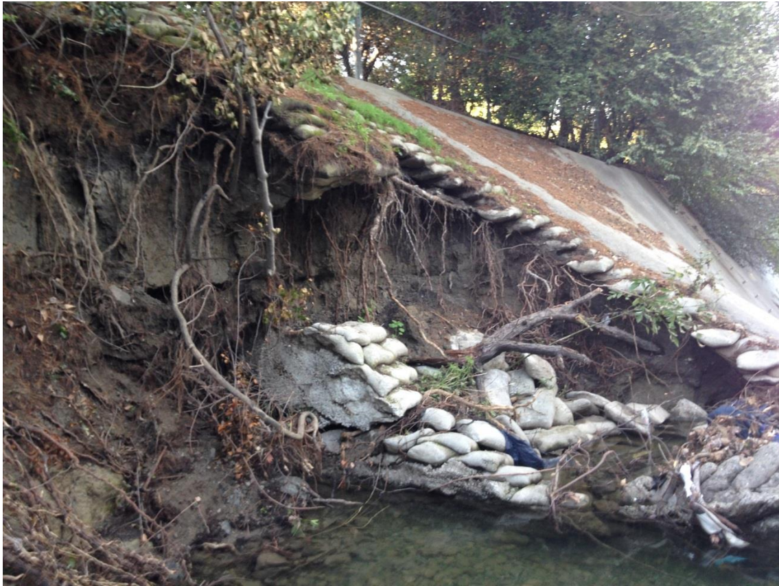
Figure 4: Heavy Erosion Located at Concrete and Earthen Channel Interface
