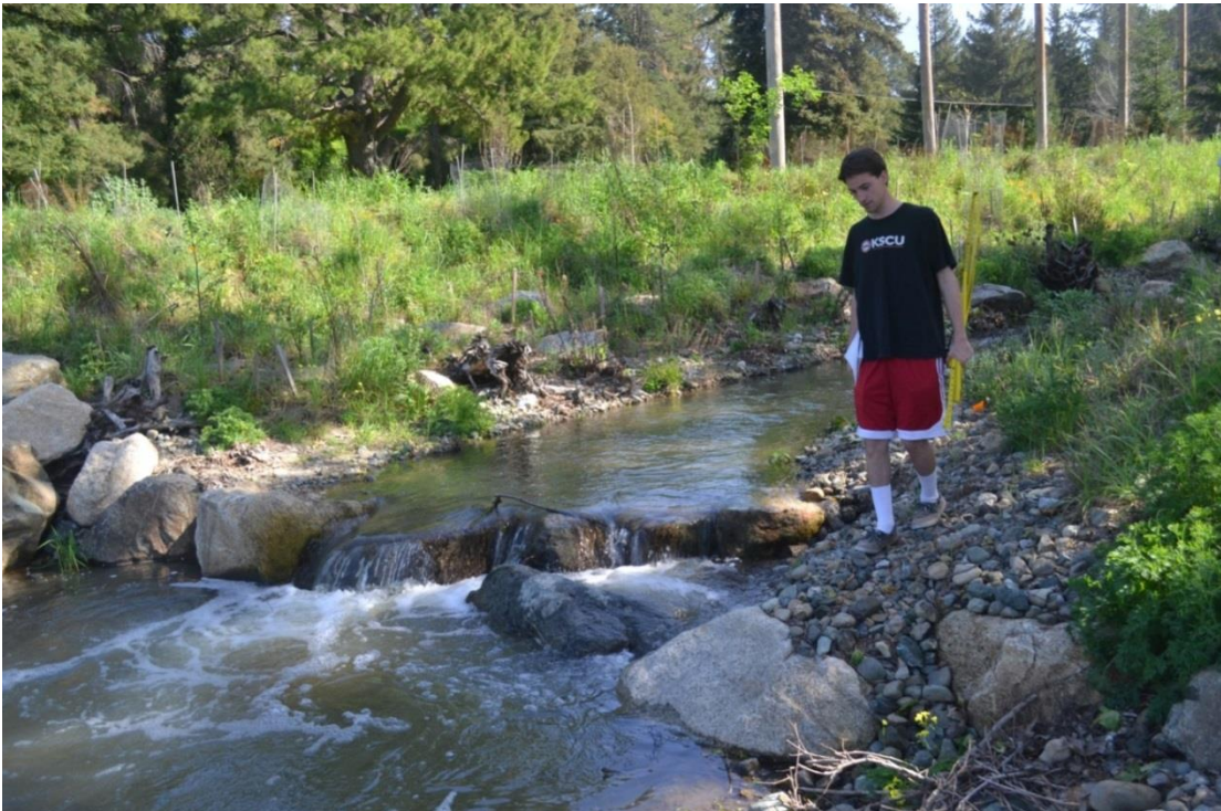
Interlocking Anchor Boulders Allow Fish to Swim Though Gaps in Rock-Promotes Fish Passage
