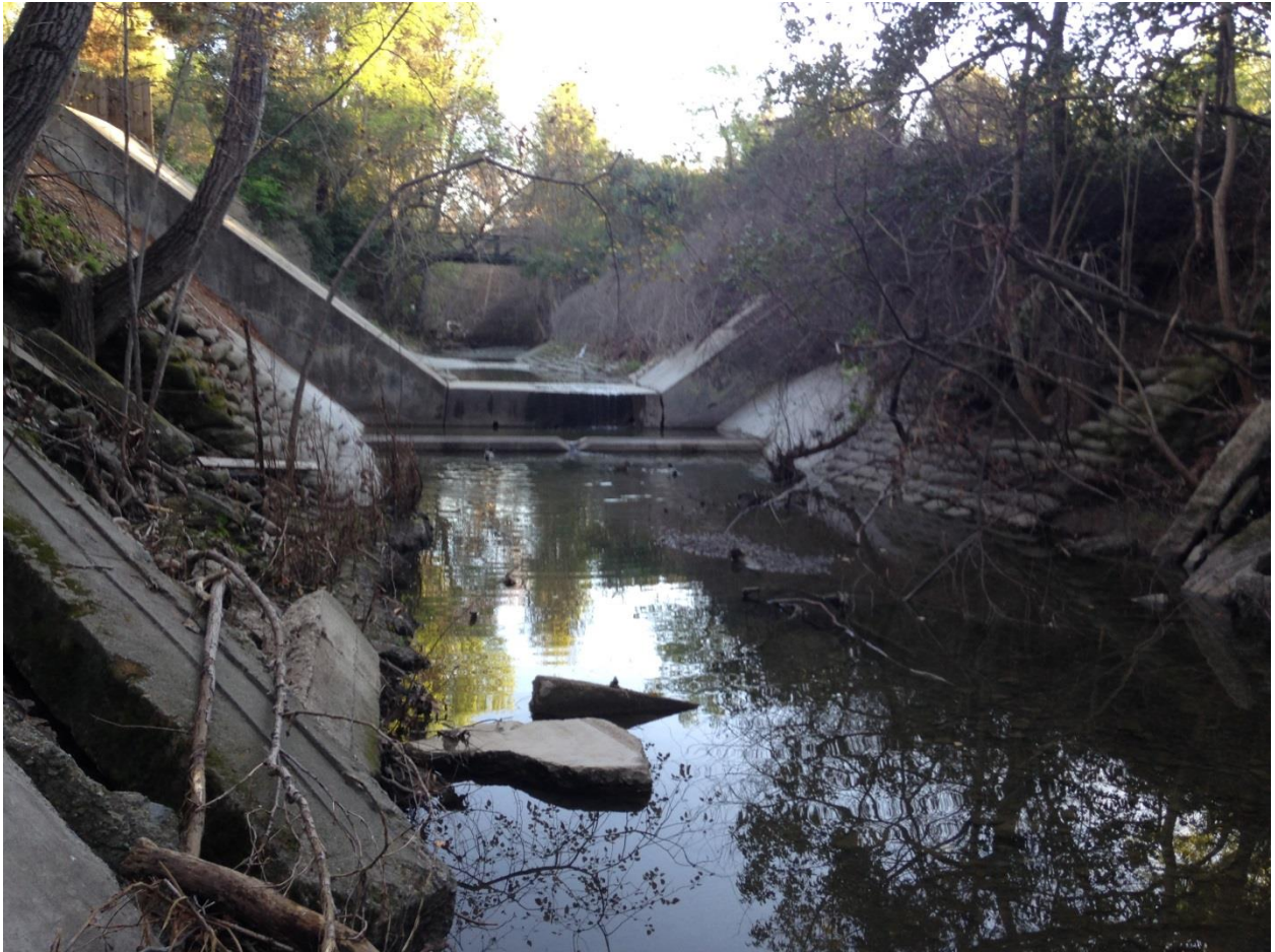
Figure 6: Hetch Hetchy Aqueduct Passage and Associated Drop a Barrier to Fish Passage
