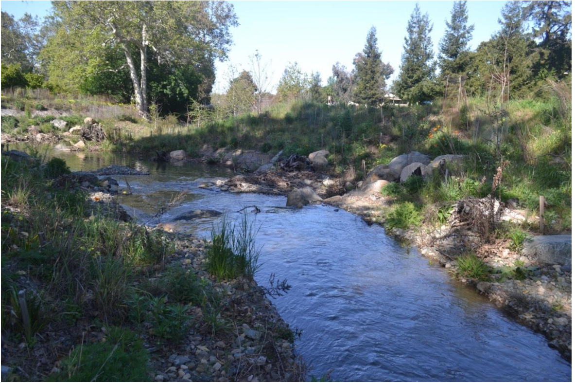
Visible Rip-Rap Embedded in Banks Increases Bank Stability and Provides Erosion Protection
