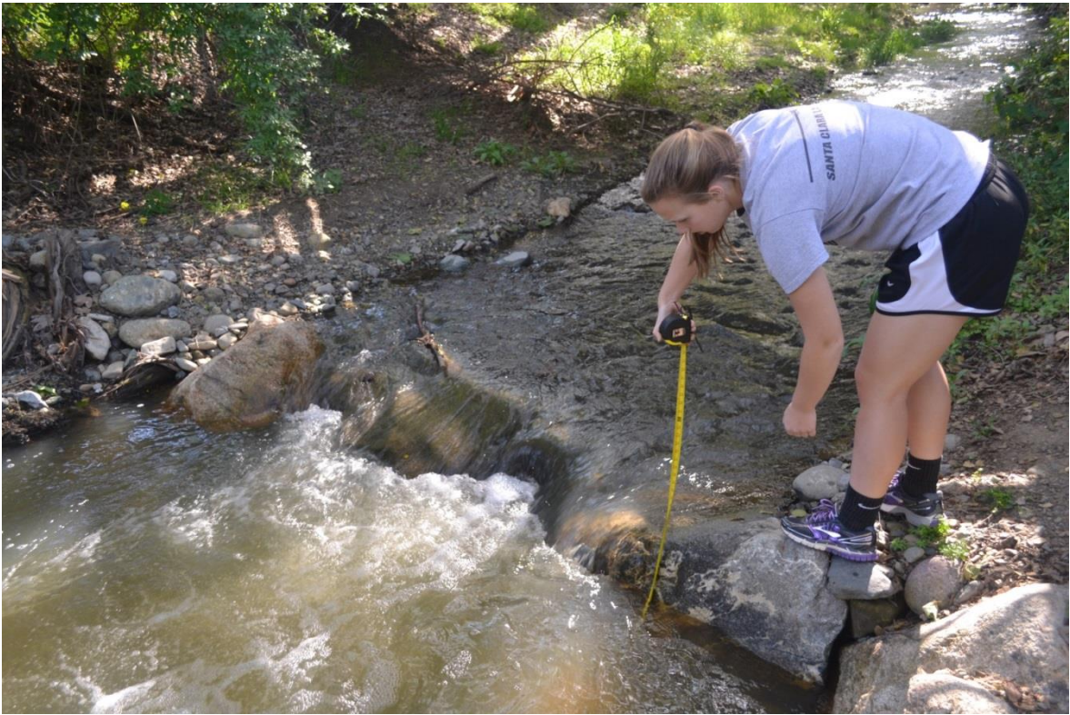
5' Anchor Boulders Secure End of Step-pool
