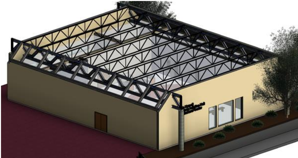
Figure 27. A 3D capture of the renovated MCC, highlighting the steel trusses.
