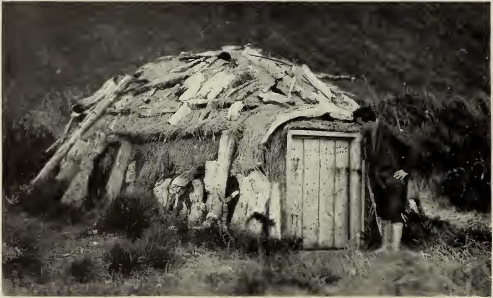
Entrance to native barabara
