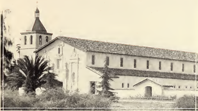
Side view. Showing in particular the roof which is covered with tile 140 years old.
