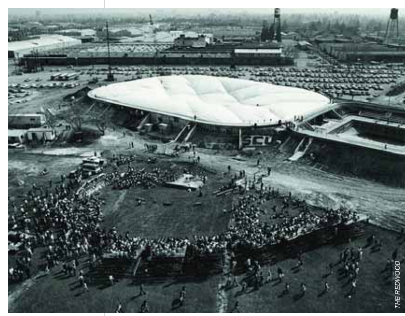
Raise the roof: With major fan support (and 11 of the big, bladed variety providing the air pressure) the Toso Pavilion bubble dome rises.
