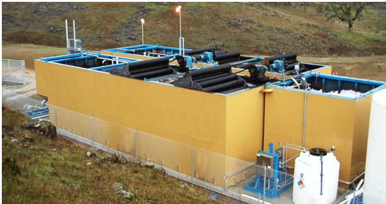
Figure 17: Common package treatment plant layout.
