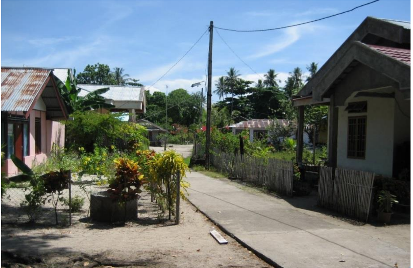
Figure 10: Higher quality concrete construction for some locals. Main road is a footpath as there are no vehicles on the island.
