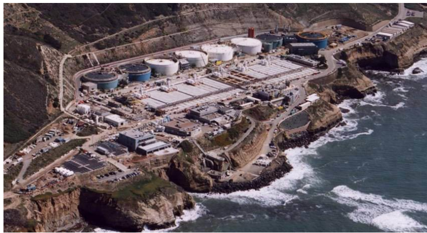
Figure 16: Municipal-Type Wastewater Treatment Facility.
