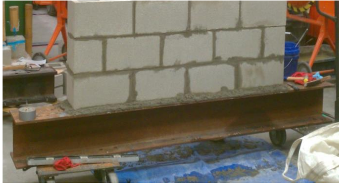
Figure 18: Steel Wide-Flange Beam Used as Strip Footing Surrogate
